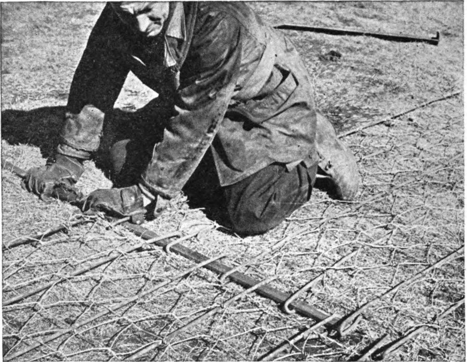
Figure 83. Method of joining Sommerfeld sections.
